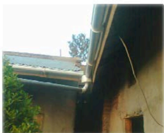
Rain water gutters connection to the water tank
